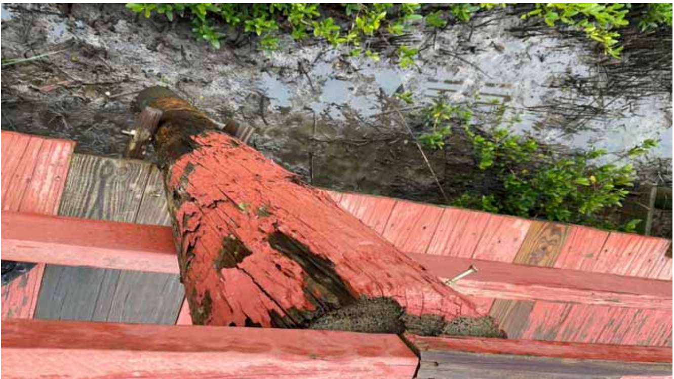
Fishing Pier Piling
