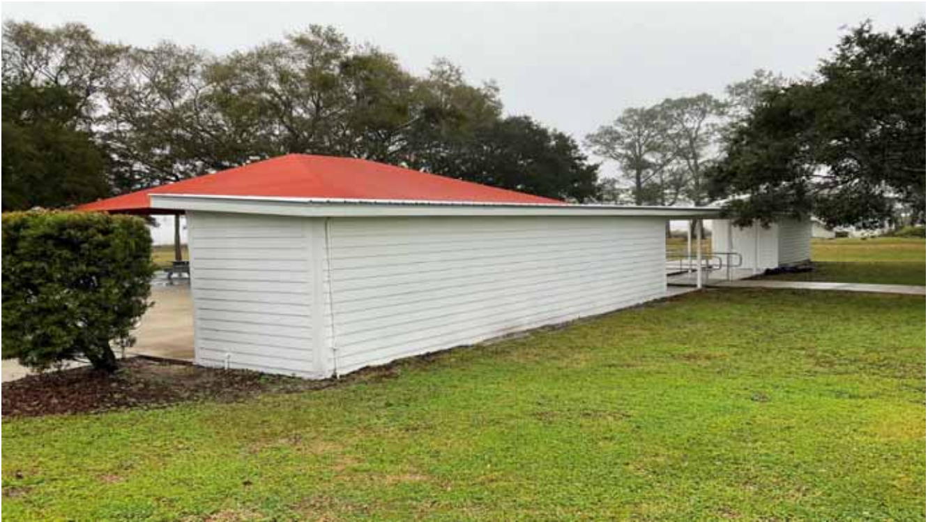
Pavilion Storage Bldg
