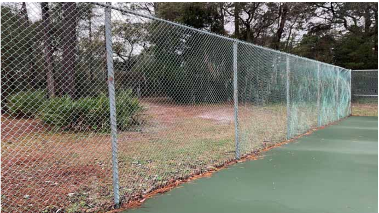
Tennis Court Fence
