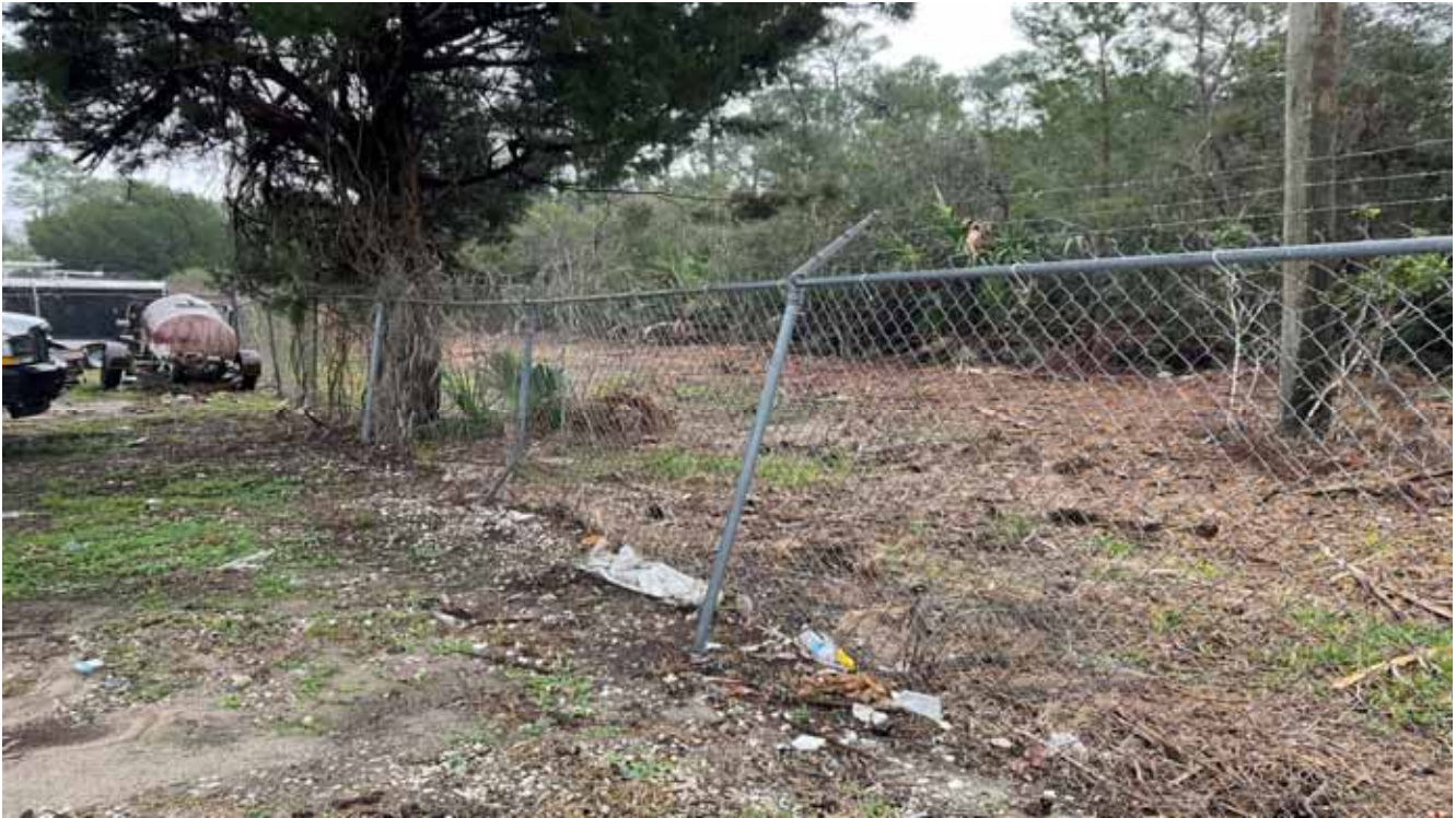
Fence - RV & Maintenance
