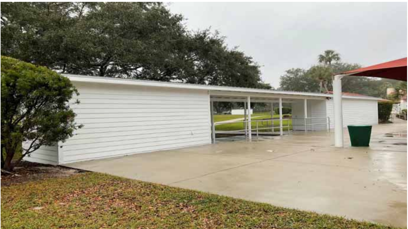
Pavilion Storage Bldg
