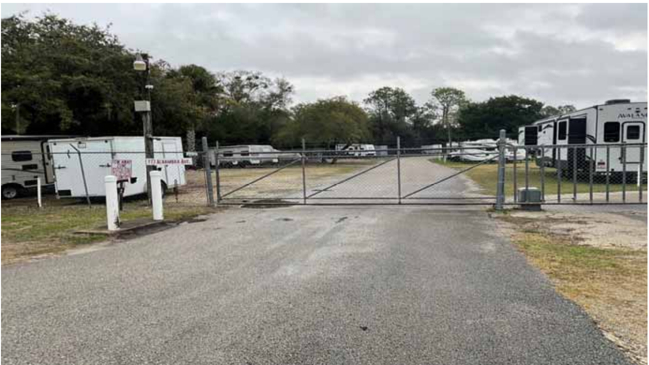
Gate - RV & Maintenance
