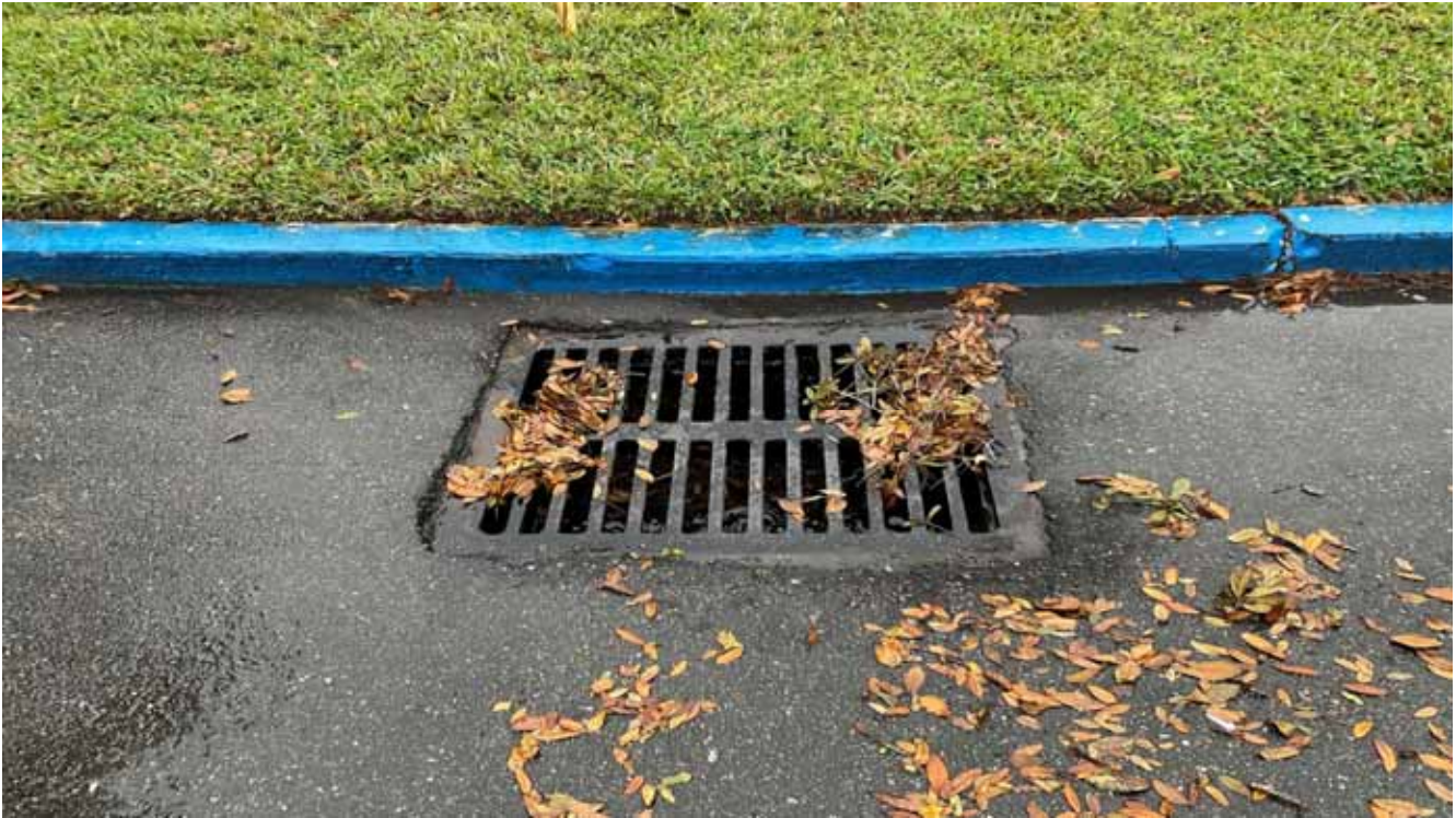
Drainage - Riverview Parking Lot
