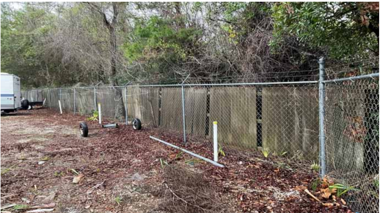
Fence - RV & Maintenance
