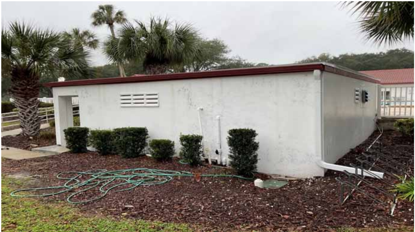
Pool Equipment Bldg
