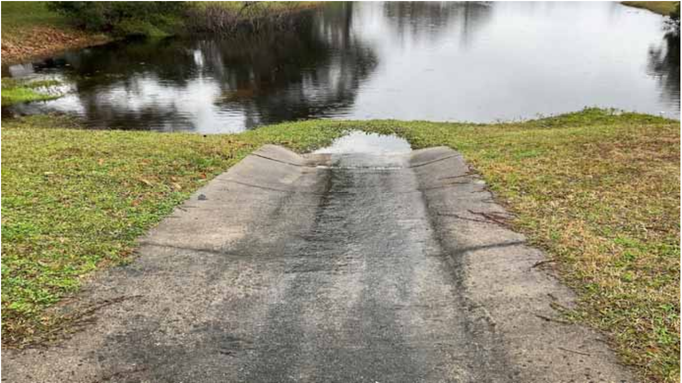
Stormwater Drainage Run-Off
