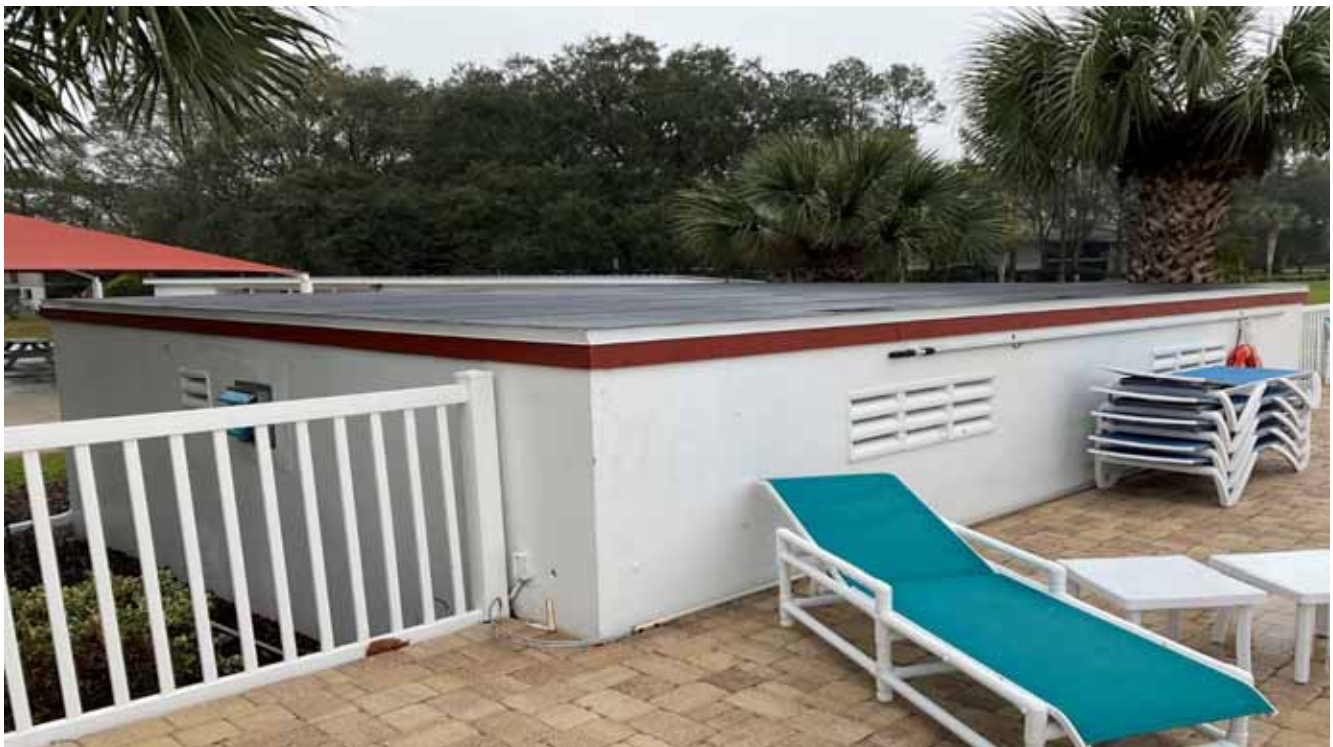
Pool Equipment Bldg
