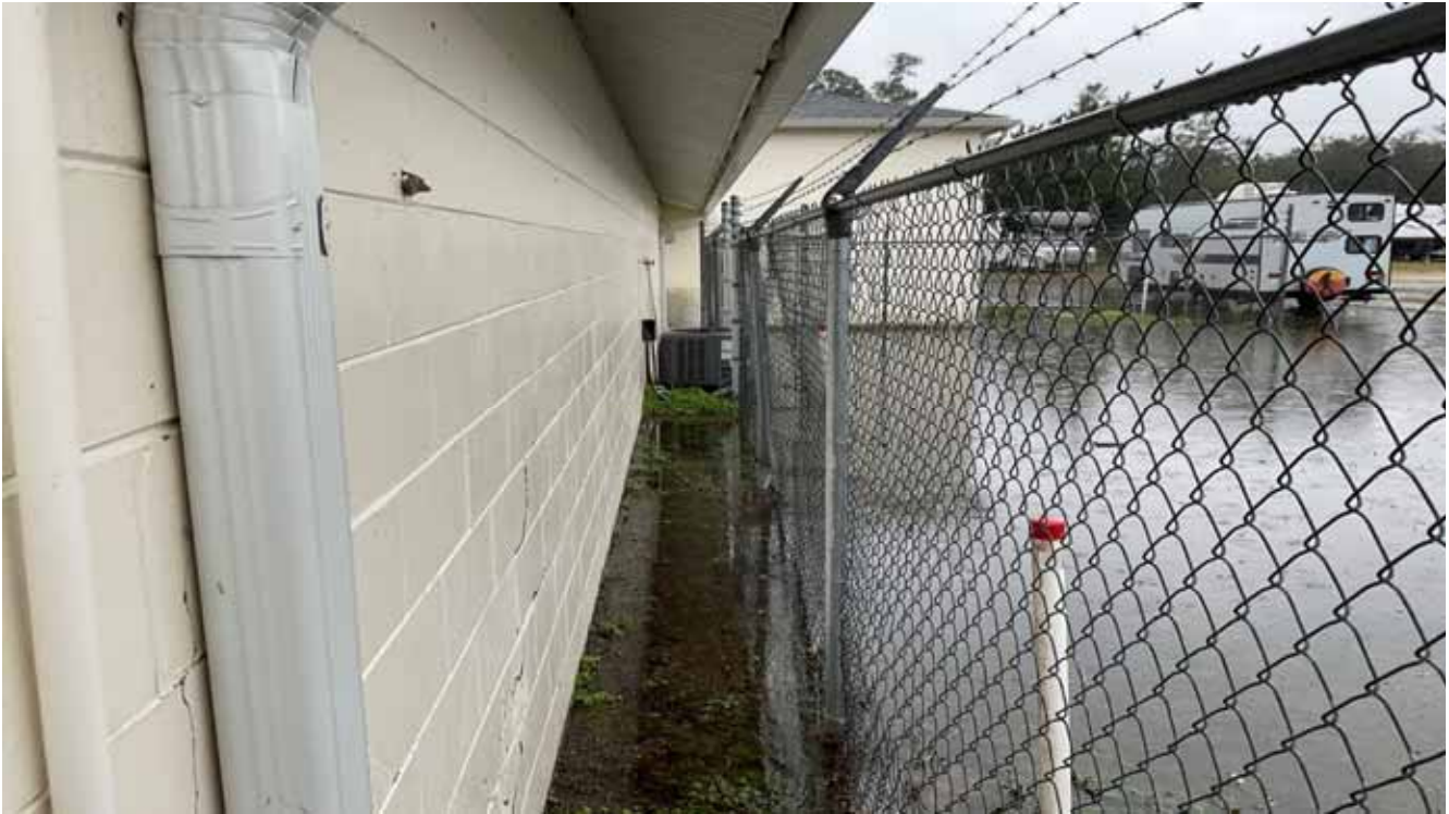
Maintenance Bldg A/C Unit
