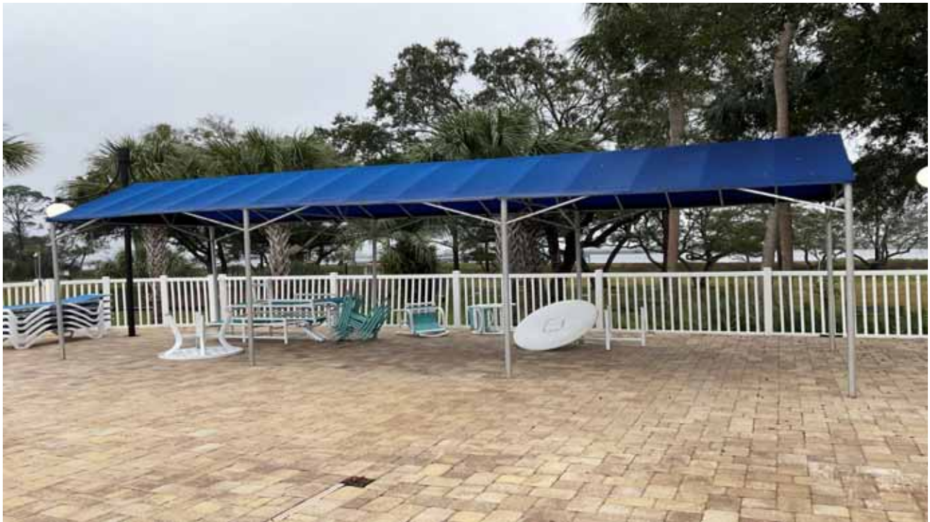
Pool Shade Structure (1 of 2)
